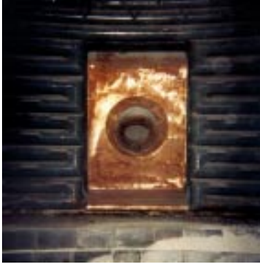
PYREJET™ nozzles are compact and easily retrofitted into existing panels.
